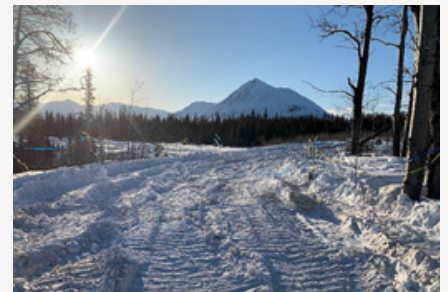
Access to the Staging and Disposal Area on the west side of the new alignment.
