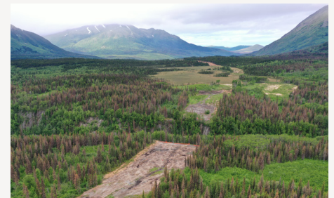
Geologists and Bridge Foundation Designers performing a site visit to the Juneau Creek Canyon. Instruments installed near the planned bridge abutments collect groundwater data from piezometers and measure for any ground movement.
