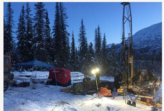
Sunrise at the West Abutment Drilling Set-up.
