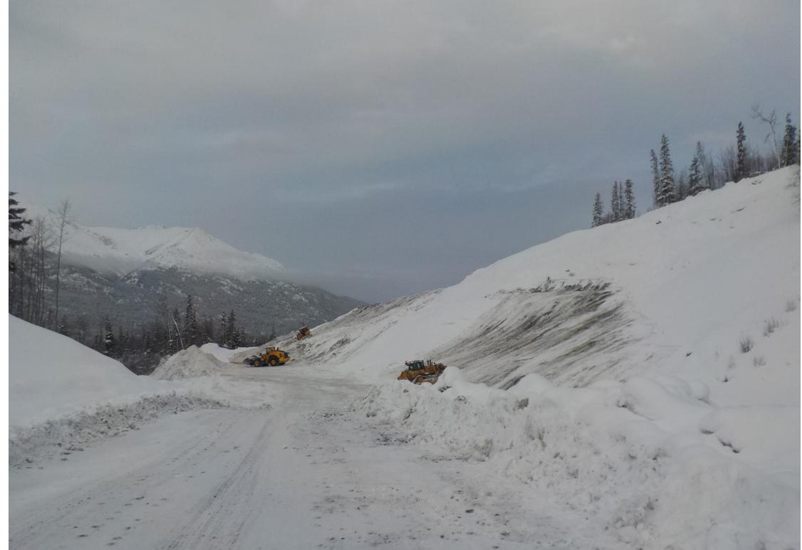
The Contractor removing snow to allow drilling and blasting activities to resume.
