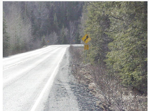
The road is narrow and curvy. Sharp curves require reduced speed.
