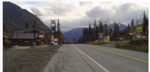
Driveways cause conflict points that slow traffic and increase the chance of crashes.
