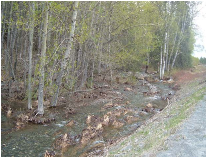
Figure 28: Drainage site D104, upstream reach showing gravel deposition.
