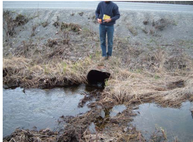
Figure 25: Drainage site D67, upstream side of existing road crossing.
