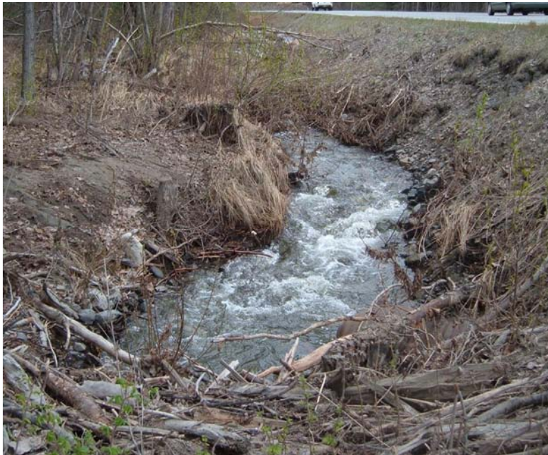
Figure 30: Drainage site D104, upstream side of existing road crossing.
