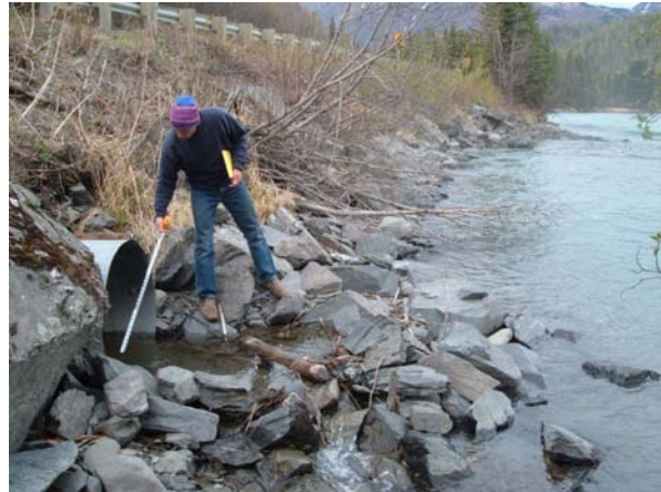
Figure 21: Drainage site D58 downstream side of existing road crossing.
