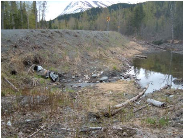
Figure 20: Drainage site D58 upstream side of existing road crossing.
