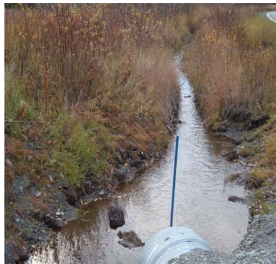
Figure 13: Drainage site D13, upstream side of Snug Harbor Road crossing.
