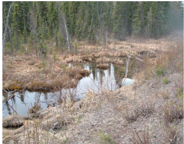
Figure 15: Drainage site D25, upstream side of existing road crossing.
