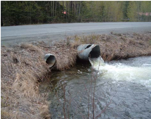
Figure 22: Drainage site D66, downstream side of existing road crossing.
