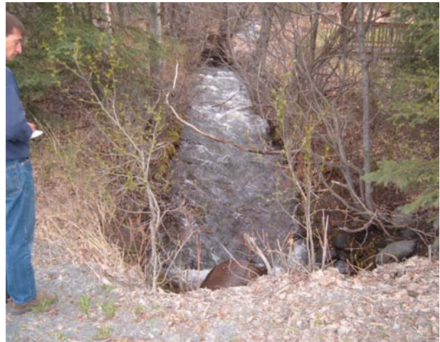
Figure 23: Drainage site D66, upstream side of existing road crossing.
