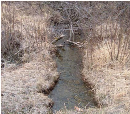
Figure 24: Drainage site D67, downstream side of existing road crossing.
