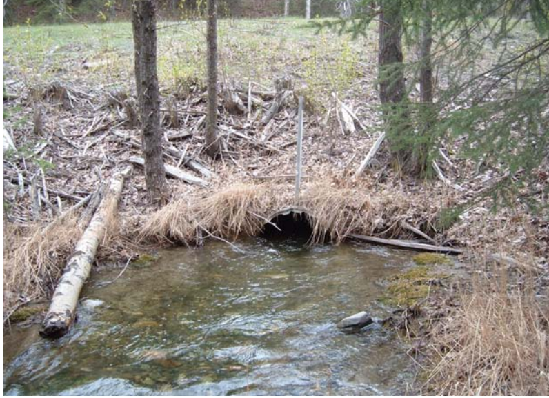
Figure 29: Drainage site D104, downstream side of existing road crossing.
