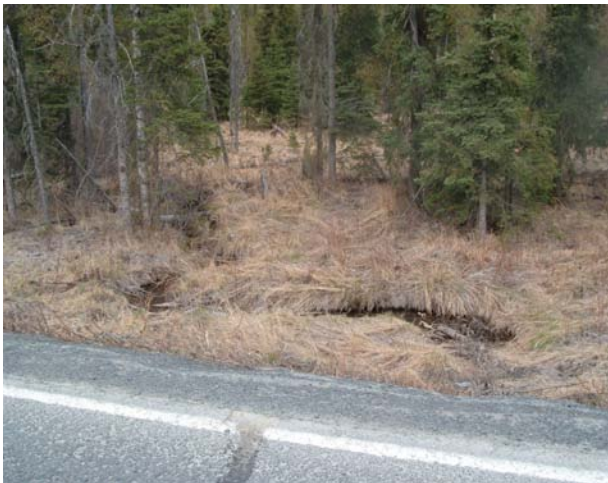
Figure 14: Drainage site D25, downstream side of existing road crossing.
